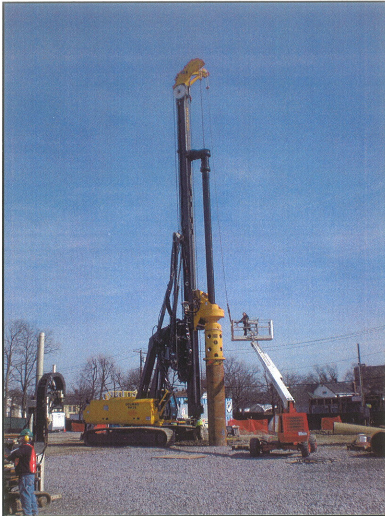
Photo 3: Delmag RH28 Drill Rig
