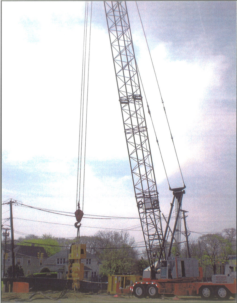
Photo 1: Pile Driving Equipment
