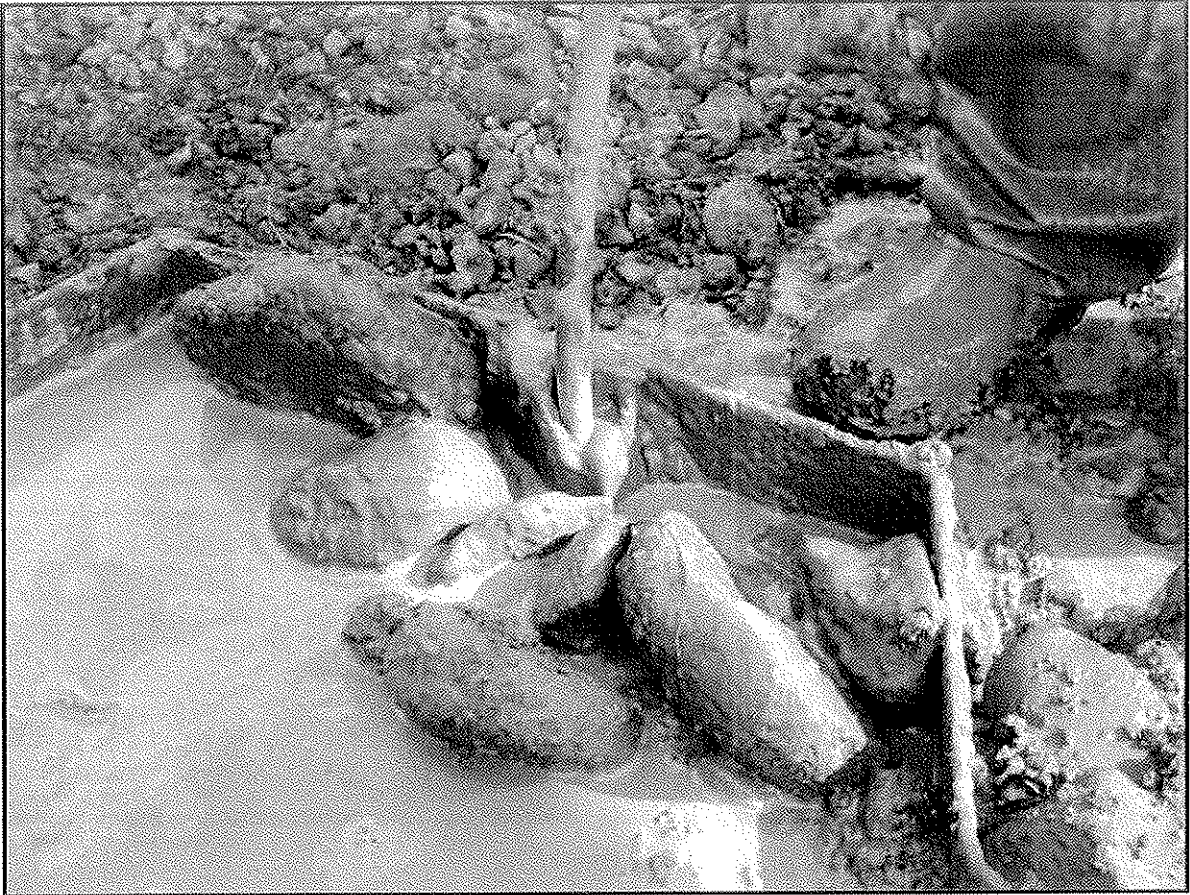
Photo 5: Typical Primary Grouting
